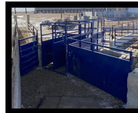
Double Chute Working Facility
